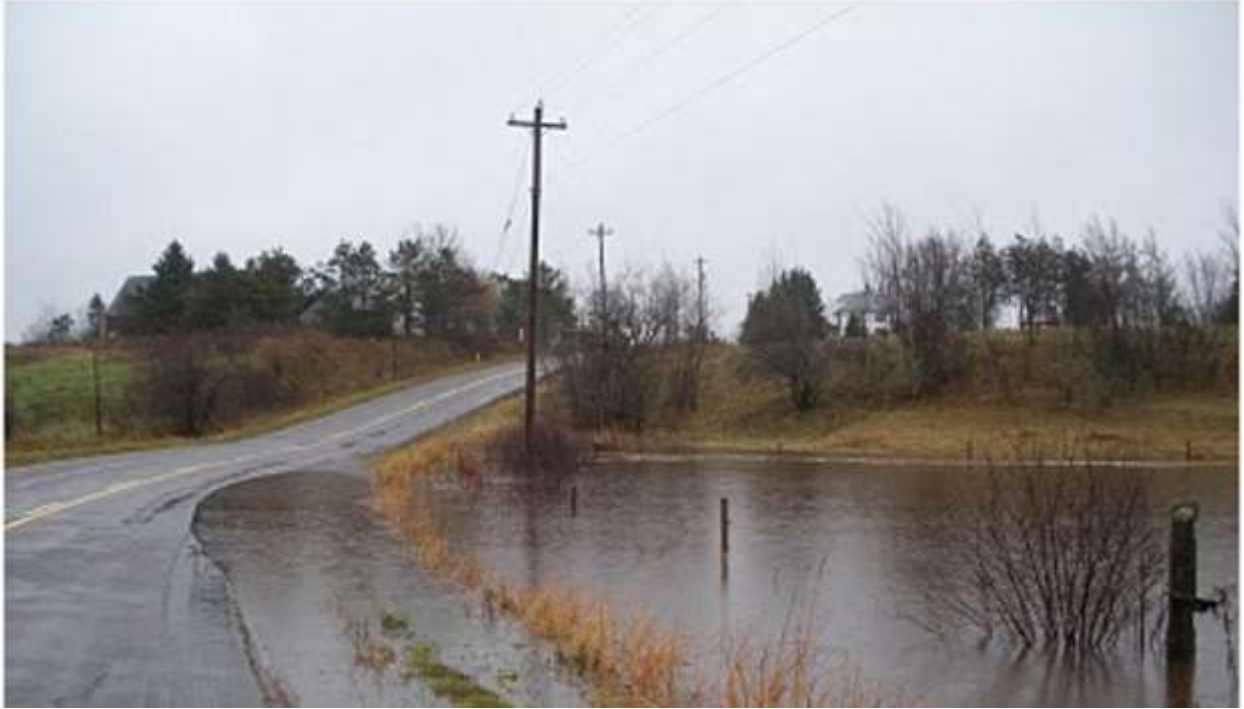
Figure 7 Smith Road was specifically targeted in this study as it was known to frequently experience a particularly high frequency of inundation. Shown here is a portion of Smith Road during such an inundation event.
