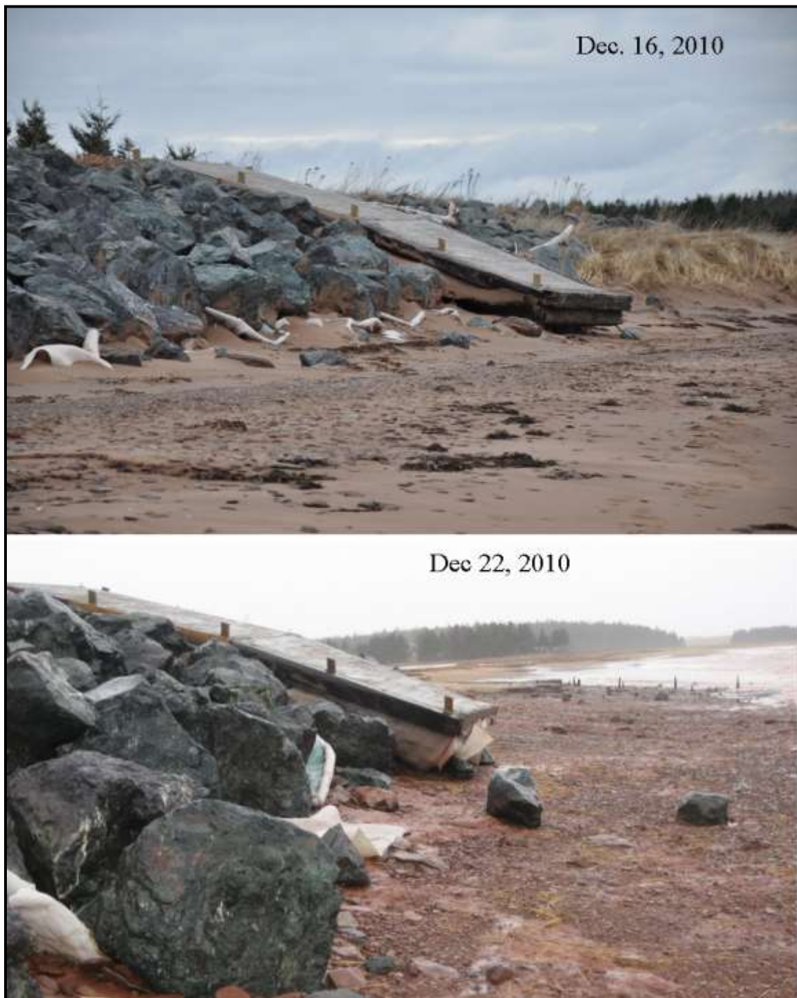
Figure 20 Erosion of the sand from the beach and destruction of the dune from the Dec. 21, 2010 storm surge event.
