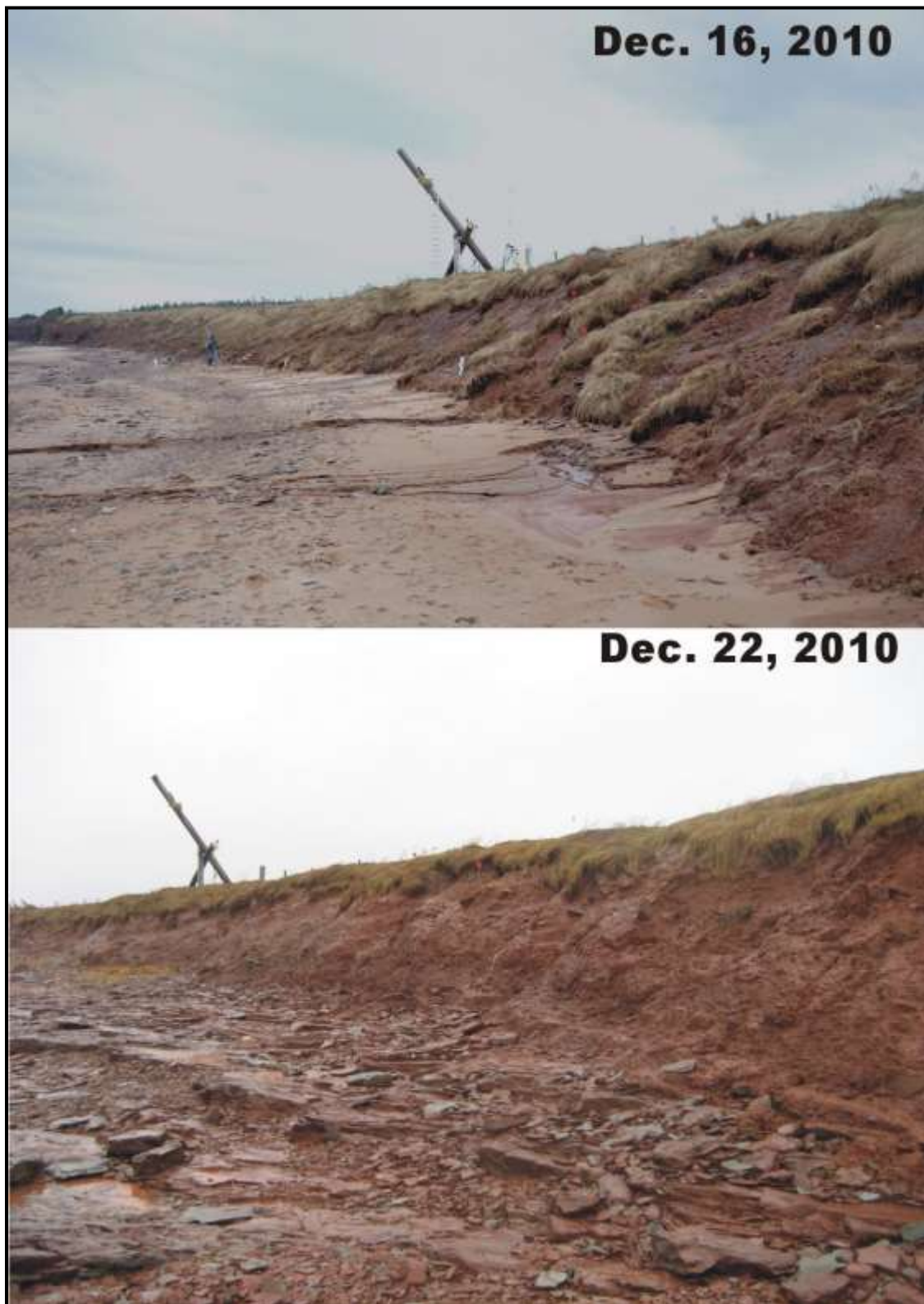
Figure 21 Erosion of the glacial till bank by the Dec. 21, 2010 storm surge event at Cape John. The pole for the time-lapse camera system and weather station are common in each photo which was taken looking east.
