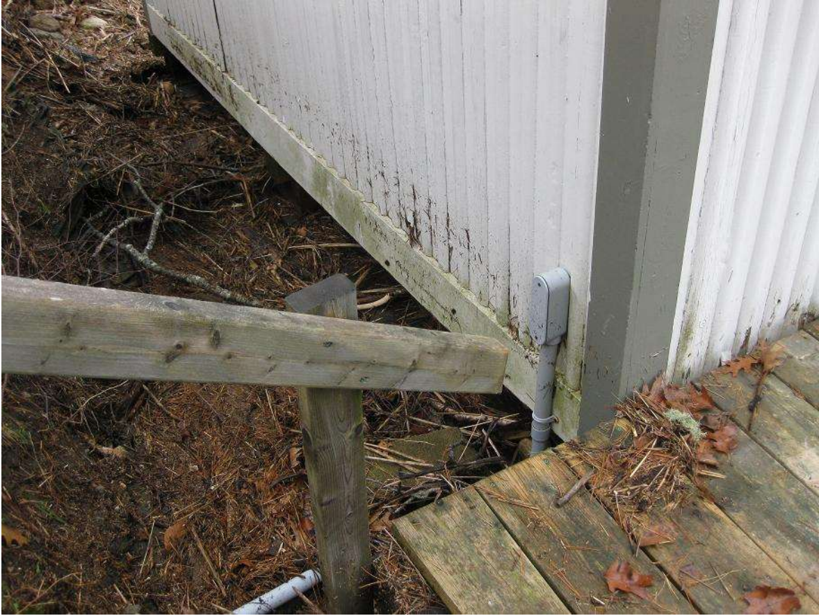
Figure 20 Upper LaHave “Mills Boat House” after Dec 6, 2010 storm surge. The debris line is marking the high-water elevation.
