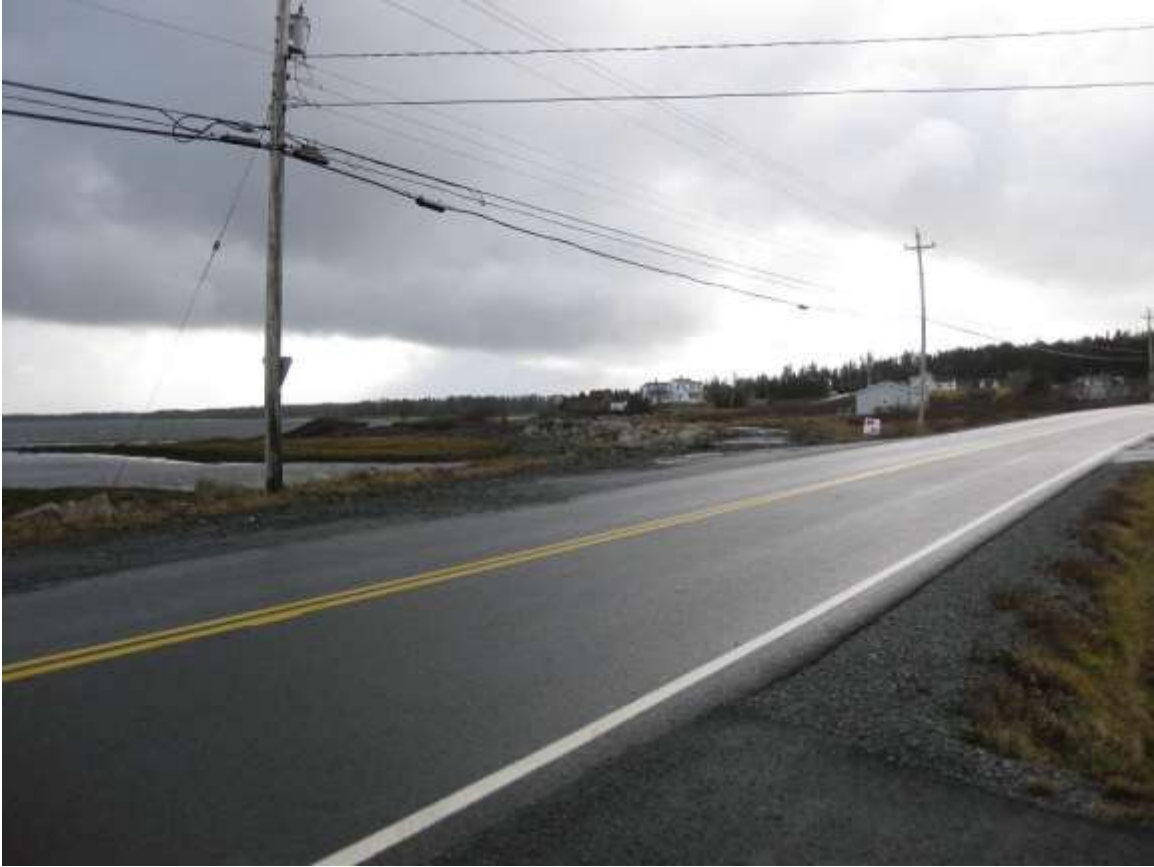
Figure 18 Dublin shore after Dec 6, 2010 storm surge. Nail in power pole marking the high-water elevation.
